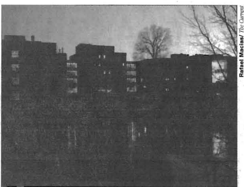
Construction of a three-phase renovation of Benton and Stadler Halls was halted after completing only the first phase because of a lack of funding.
